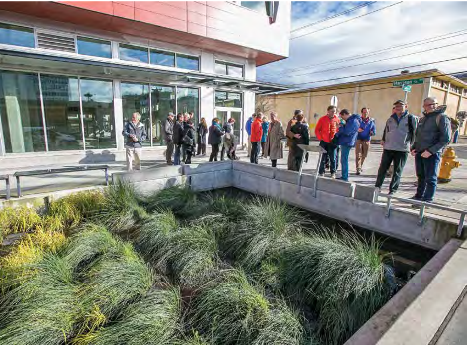
Stormwater Bioswale. Seattle, WA. © Paul Joseph Brown
