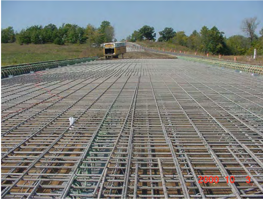
Figure 1. Stainless Steel Reinforcement of Bridge A6059
