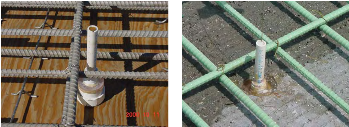
Figure 2. Sensor Housings Installation
