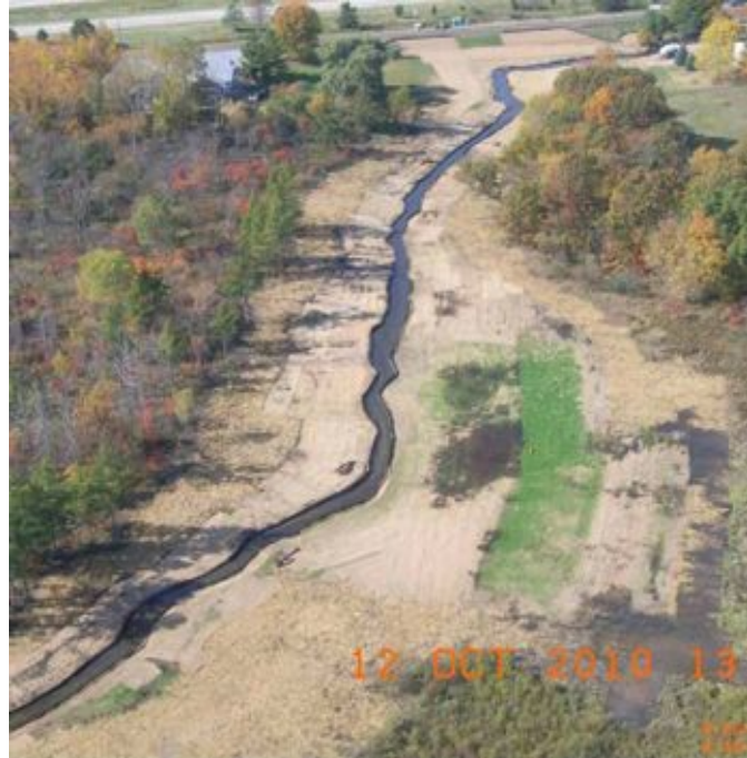
Insert 4-4 Talmadge Creek shortly after mat roads were removed near MP 1.00.
