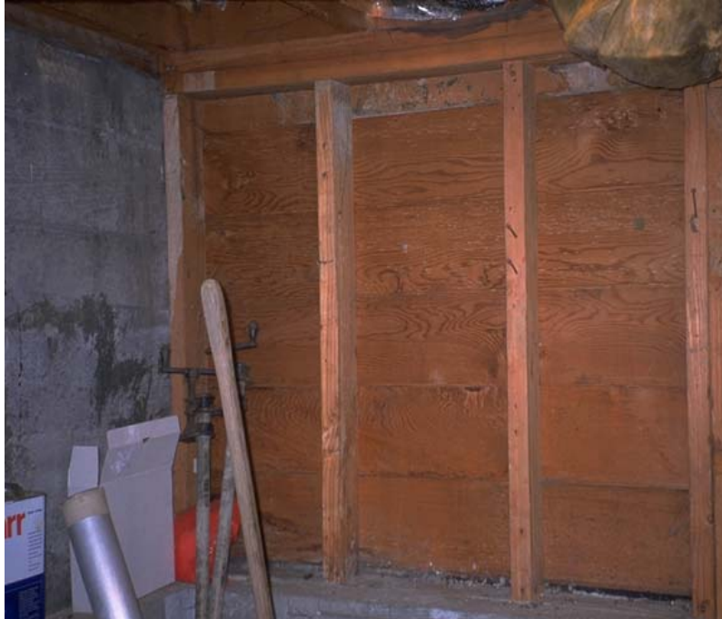
Figure 9 A pony wall without structural panels which are needed to strengthen it to resist excessive side sway. (Photo by Tom Hall)
