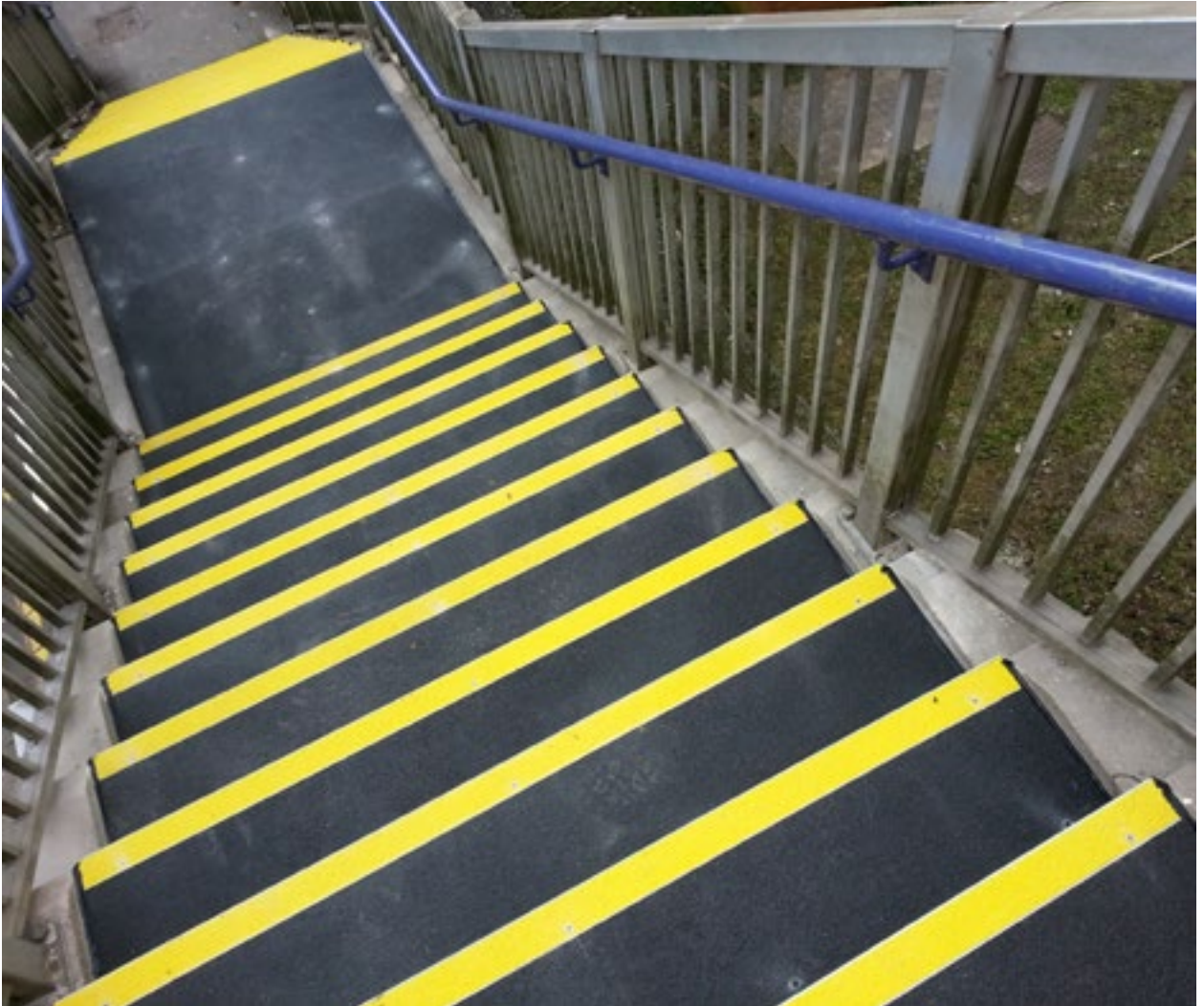
Figure Q1.1 A typical station footbridge staircase
