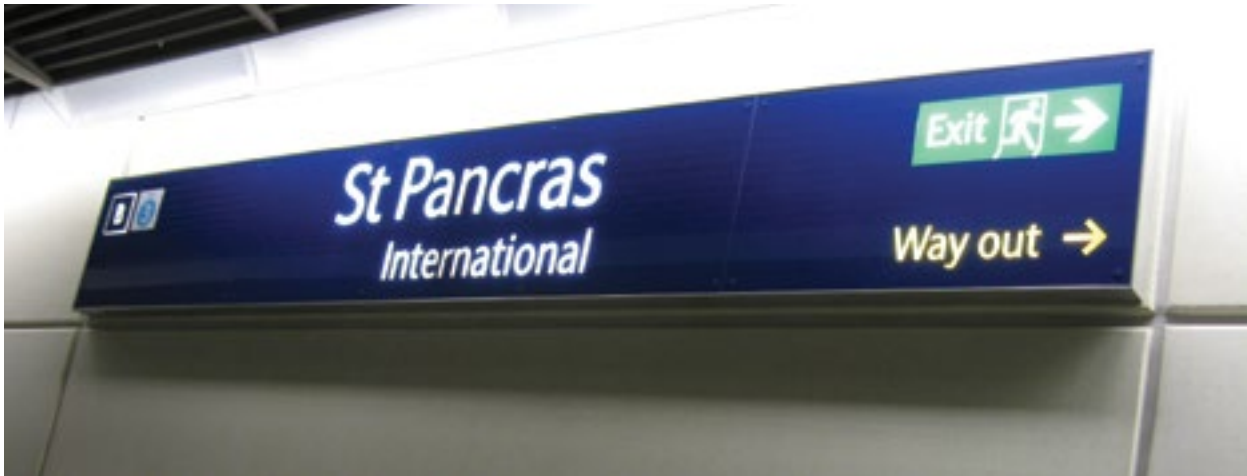
Figure K5.1 Example of a backlit platform sign
