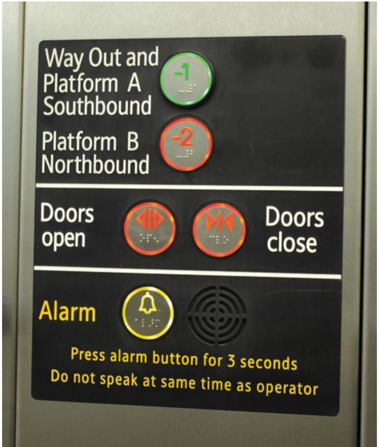
Figure K6.1 Lift control buttons with braille markings
