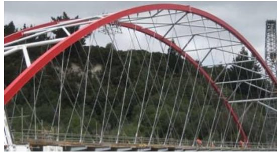
Figure 148 – Example of an efficient bracing system. Waikato River Network Arch Bridge.
