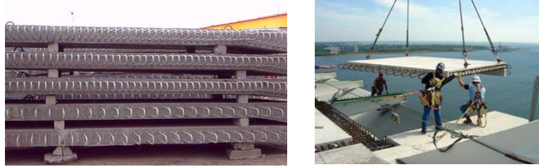
Figure 52 – Precast concrete slab solution examples.
