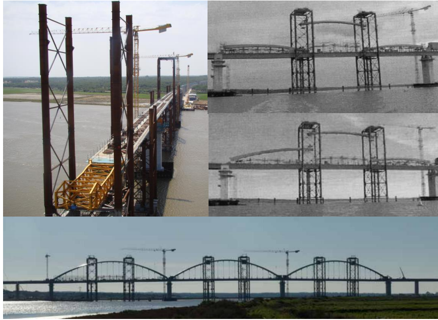
Figure 48 – New Sado Railway River Crossing.
