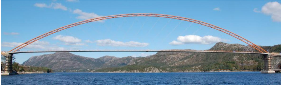
Figure 8 - The Brandanger Sound Bridge - by Per Tveit . 220 m Span
