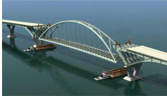
Figure 45 – Arch being lifted into position by small cranes over the approach spans. Lake Champlain Bridge (2011).
