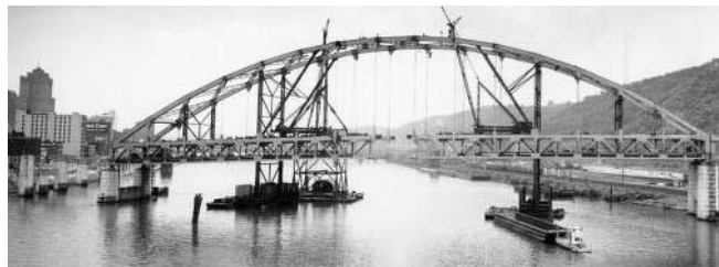
Figure 46 - The Fort Pitt Bridge (1959), during its construction phase.
