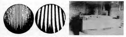
Figure 2. Left: the light-interference fringes as seen in the interferometer telescope, fringes shifted laterally as the instrument was rotated. Right: the original Michelson-Morley interferometer with an approximate 22-meter round-trip light-beam path, mounted on a concrete platform in the basement of the old Case School Physics building.
