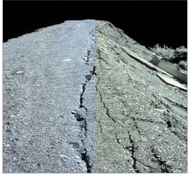
➤ FIGURE 8: LONGITUDINAL CRACKING Regular surveillance inspections can spot issues such as longitudinal cracking so they can be addressed or reported promptly.
