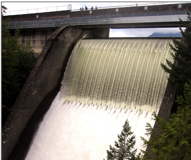
📍 The CLEVELAND DAM in North Vancouver is a concrete dam that supplies about 40 per cent of the Lower Mainland's fresh drinking water.
