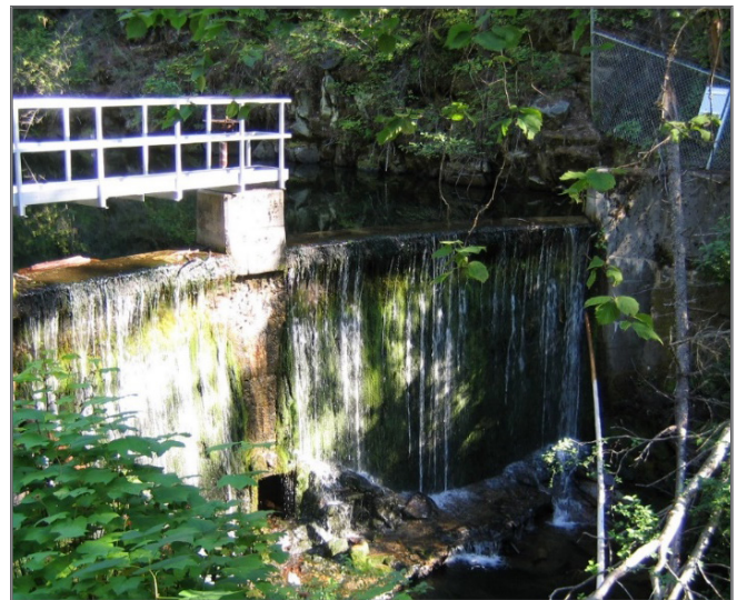
📍 SMOKY CREEK DAM, a small concrete dam near Nelson
