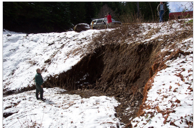
➤ FIGURE 8: LONGITUDINAL CRACKING Regular surveillance inspections can spot issues such as longitudinal cracking so they can be addressed or reported promptly.
