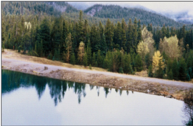
FIGURE 15: Shows a well-maintained dam
