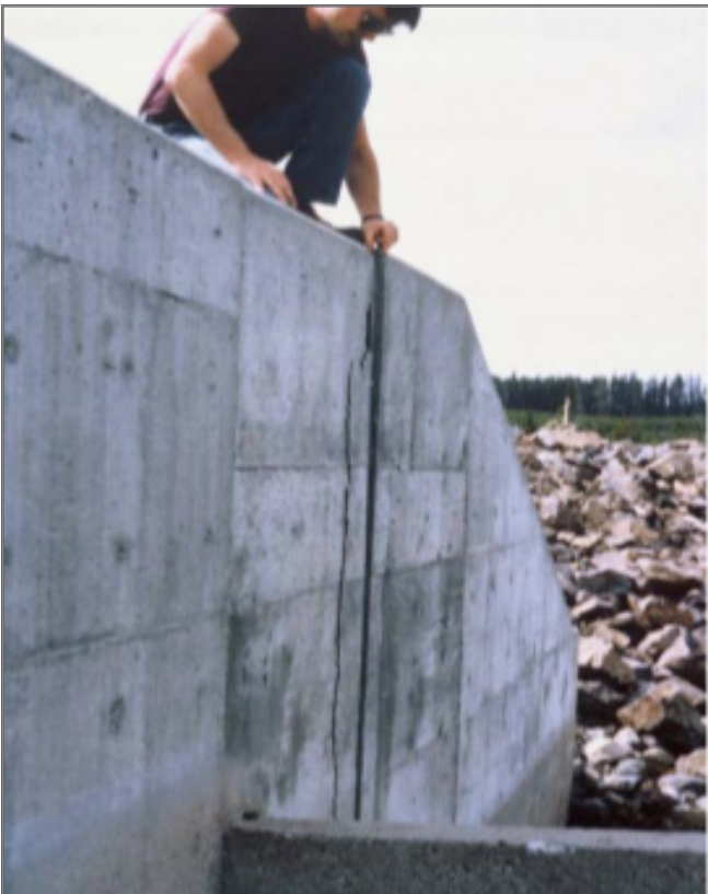
FIGURE 11: Inspecting a spillway training wall
