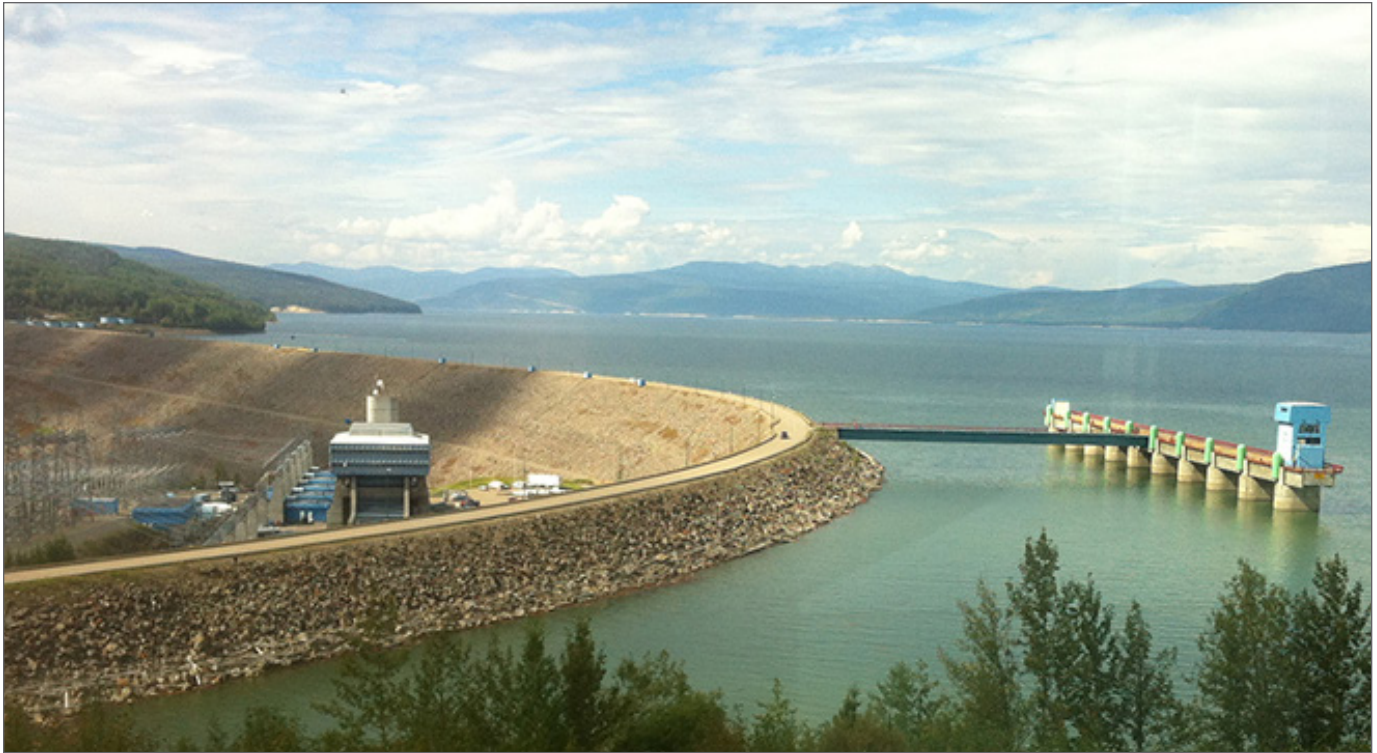
📍 The W.A.C. Bennett Dam in northwest B.C. is as high as a 60-storey building and two kilometres long, and holds back the 360 kilometres of Williston Lake, the largest reservoir in North America.
