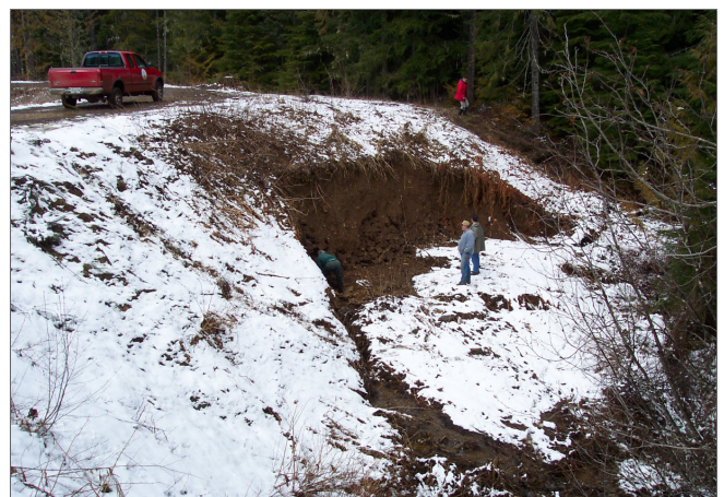
➤ FIGURE 9: Dam sloughing caused by longitudinal cracking and vertical displacement
