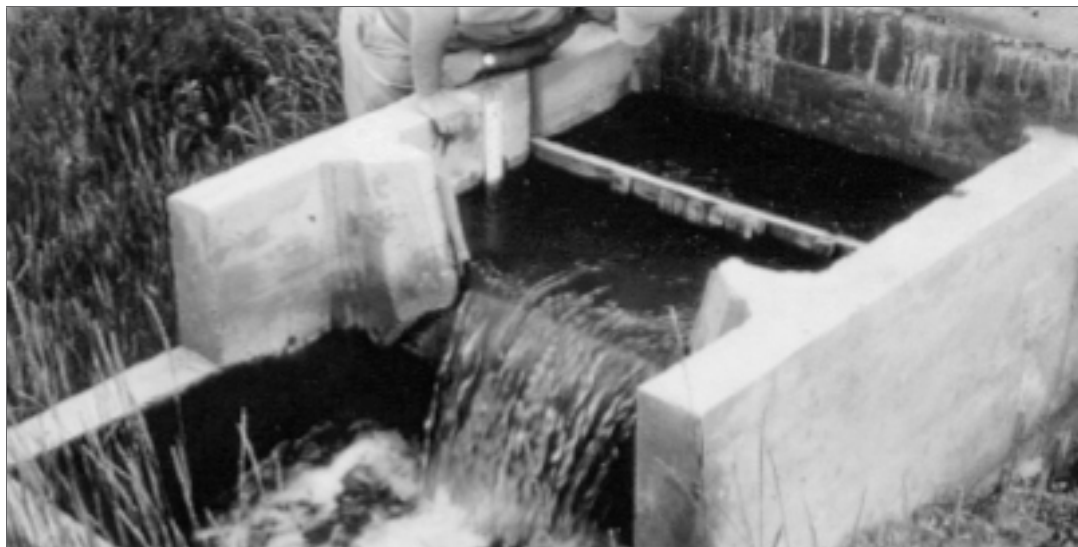
🔗 FIGURE 17: Outlet discharge weir
