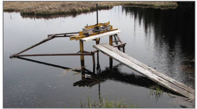
FIGURE 12: Typical outlet gate valve
