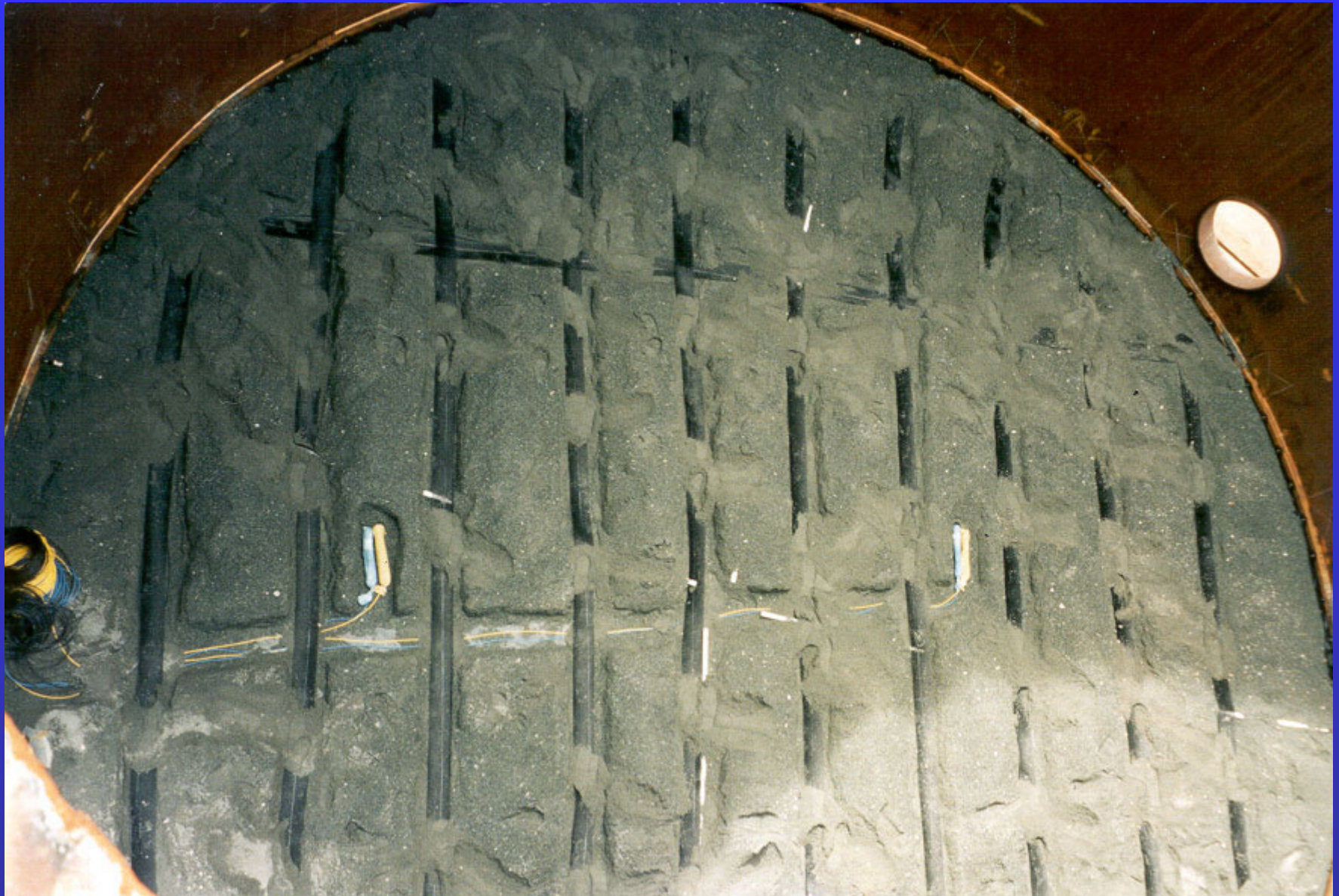
CP Installation on Rebottomed Tank
