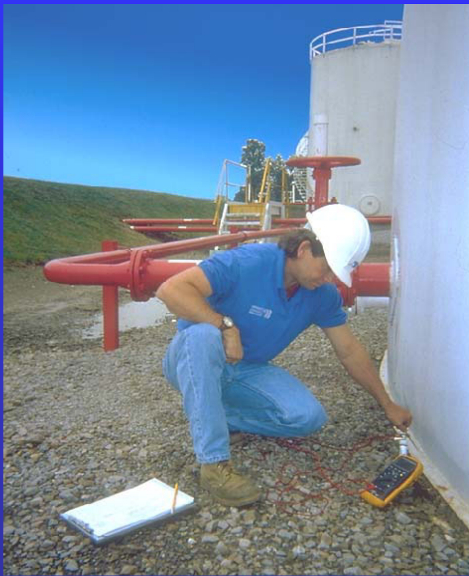
Cathodic Protection Monitoring
