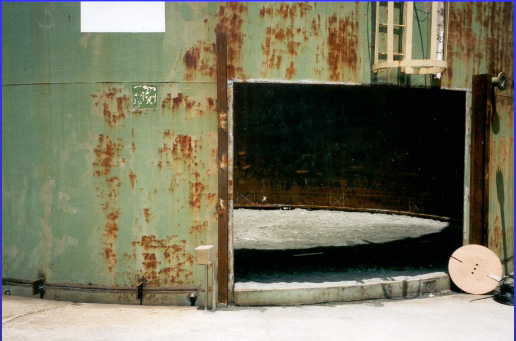
New Floor Installation on Existing AST
