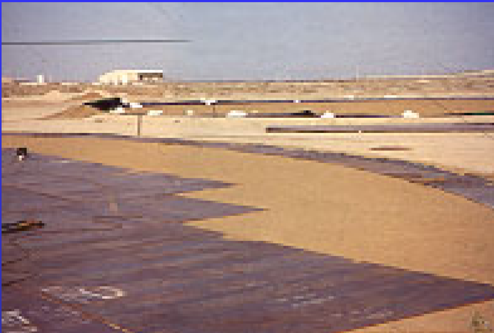
Floor Plate Installation
