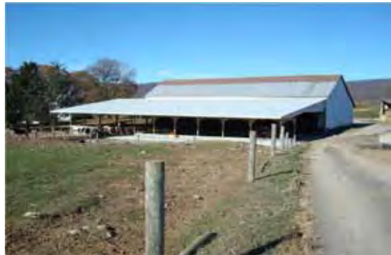
After: Implemented roof and heavy use area.
