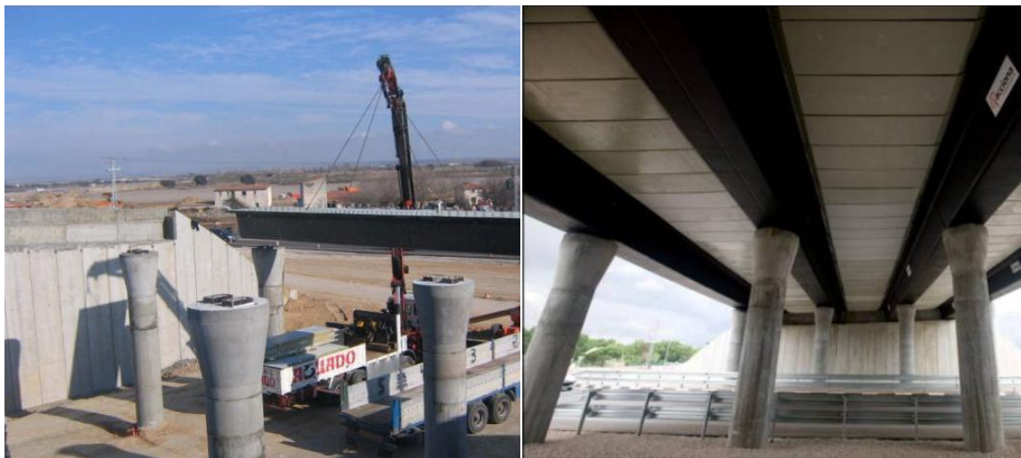
Figure 5 Bridge with FRP deck during construction and after compilation.
