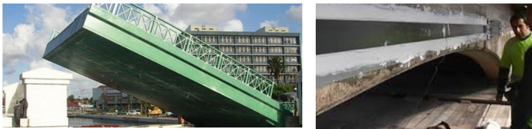
Figure 1 FRP bridge and strengthening and repair of bridges. Figure sources: GEF Company, Tenroc Company.
