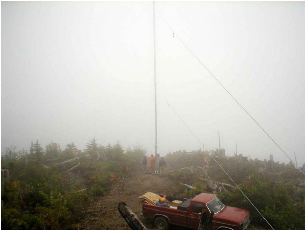
Figure 7, MCB Site with Tower
