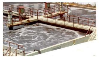
Fig 2. : Ejector aerator in the equalization tank
