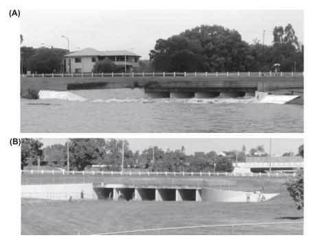
Fig. 9. Minimum energy loss culvert along Norman Creek beneath Ridge Street, Brisbane (Australia). (A) Inlet operation on 7 Nov. 2004 for  $Q \approx 80$  to 100 m<sup>3</sup>/s; (B) Outlet on 13 May 2002.
