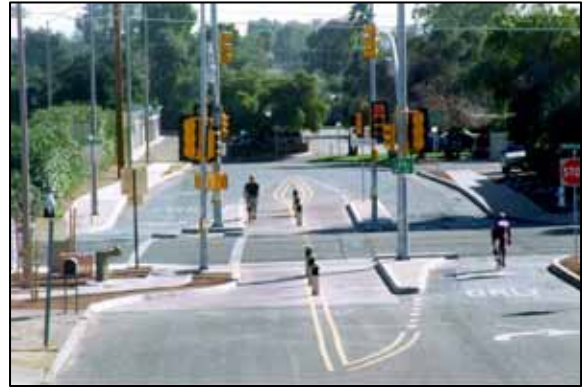
Figure 11.11 - Toucan Signal in Tucson, Arizona (Photo by Richard B. Nassi)
