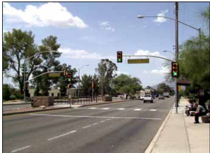
Figure 11.10 - Pelican Signal in Tucson, Arizona (Photo by Richard B. Nassi)
