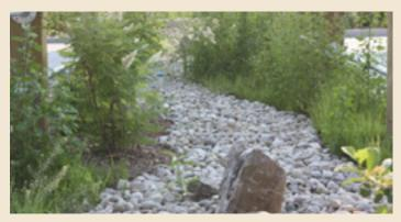
A bioswale captures stormwater run-off from the parking lot.
