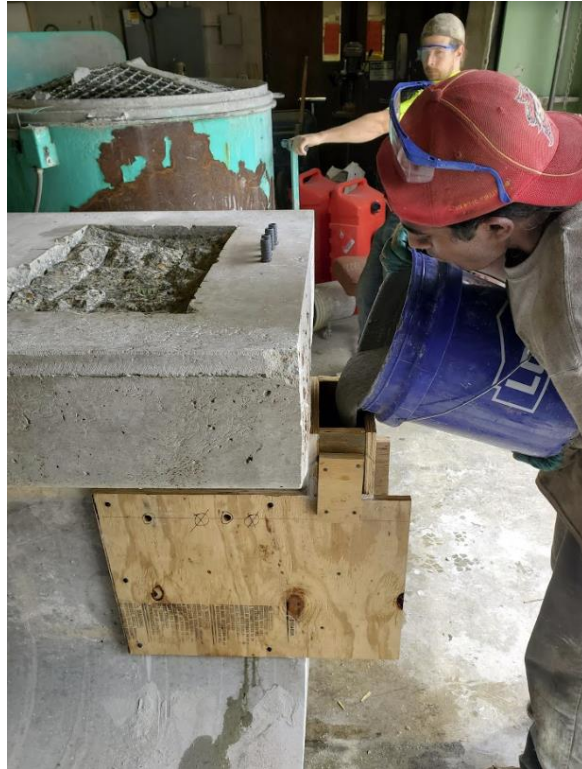
Figure 4.8. Patch mix being poured into formwork
