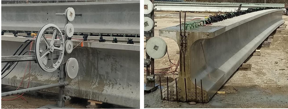
Figure 4.2. Wire saw cutting in progress
