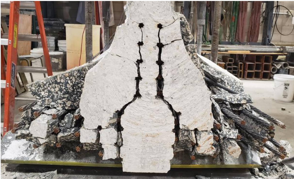
Figure 4.15. South beam end of Control-2 after failure
