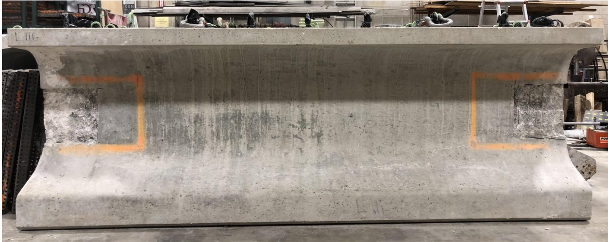
Figure 4.6. Artificially damaged beam specimen (1 ft damage)
