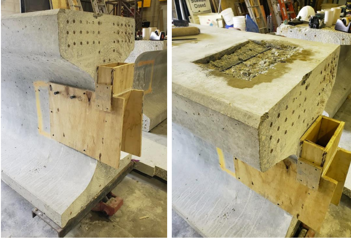
Figure 4.7. Beam patching formwork (left) and wetted area to be patched (right)
