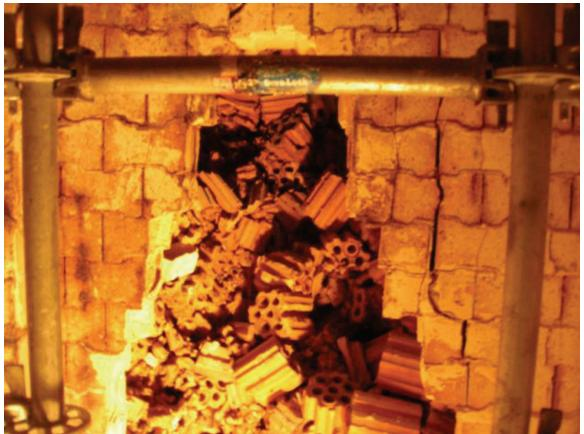
Figure 2: The hole in the partition wall
