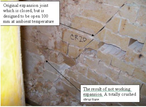
Figure 4: The compromised Xmas tree expansion joint design under the Dome
