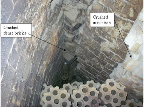
Figure 3: The crushed corners
