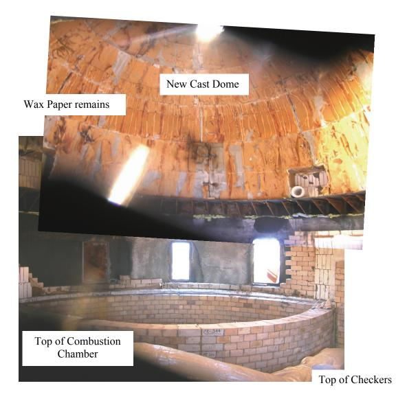
Figure 8: The cast dome supported and the Walls coming up.
