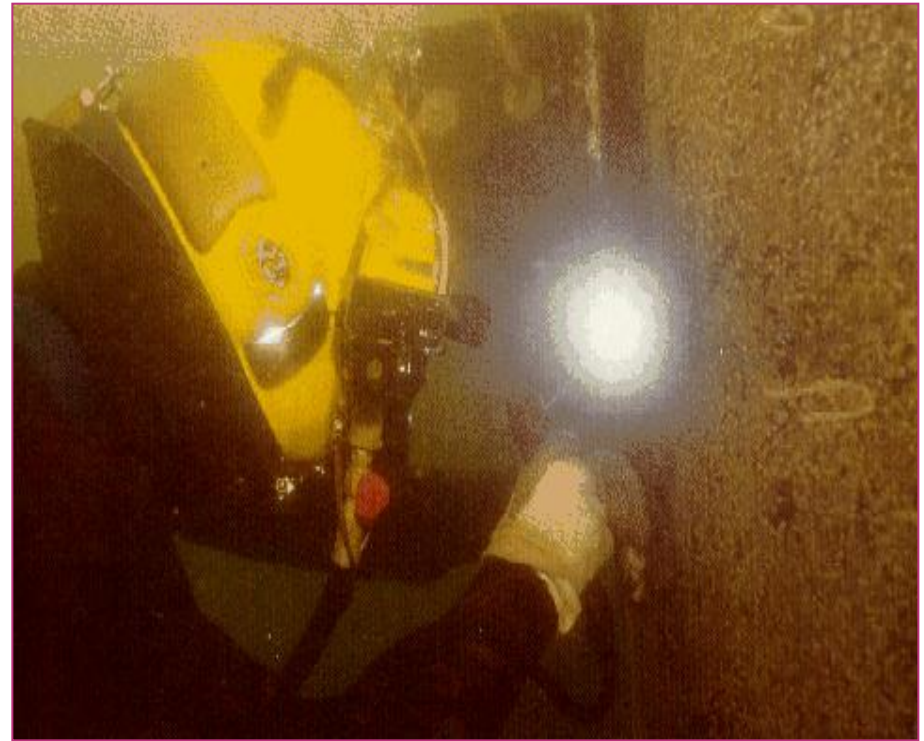
Underwater welding with SMAW
