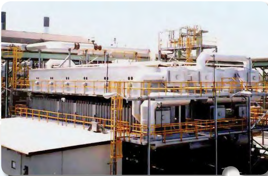
At 11.2 MGD, this Multi Stage Flash installation on the island of Aruba is one of the largest in the Caribbean and guarantees quality water for all the island's needs. In fact, Aruban drinking water has been dubbed "the champagne of the Caribbean," and is even bottled and shipped to nearby Curacao.
