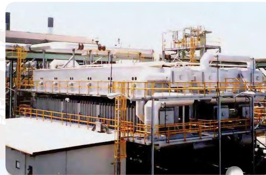
At 11.2 MGD, this Multi Stage Flash installation on the island of Aruba is one of the largest in the Caribbean and guarantees quality water for all the island's needs. In fact, Aruban drinking water has been dubbed "the champagne of the Caribbean," and is even bottled and shipped to nearby Curacao.
