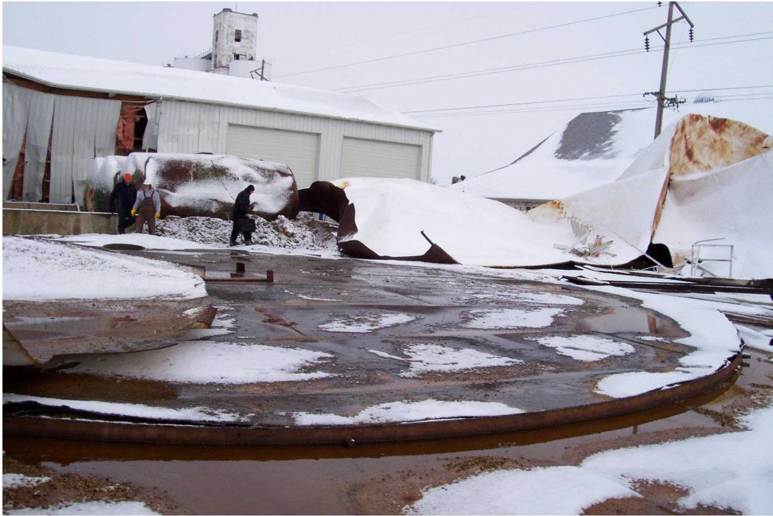
Original tank foundation
