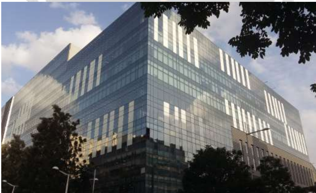
Figure-3.4 Exterior View of Mfar Philips, Bengaluru
