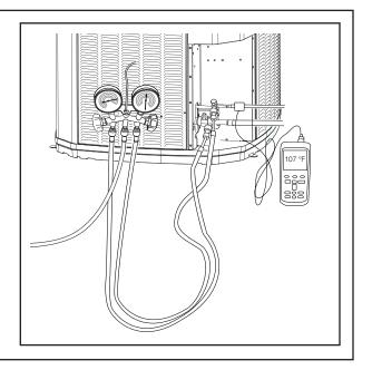
Use the liquid line temperature and liquid line gage pressure from Step 2, along with the Dip Switch setting column, to determine the proper Liquid Gage Pressure.
