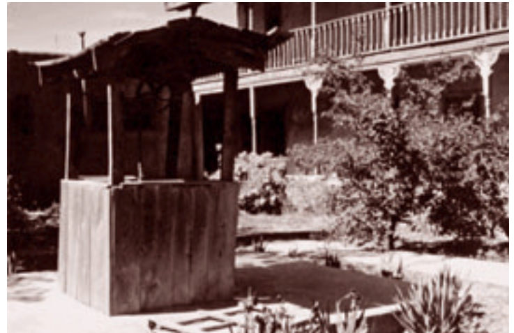
COURTYARD OF THE HOUSE, n.d.
