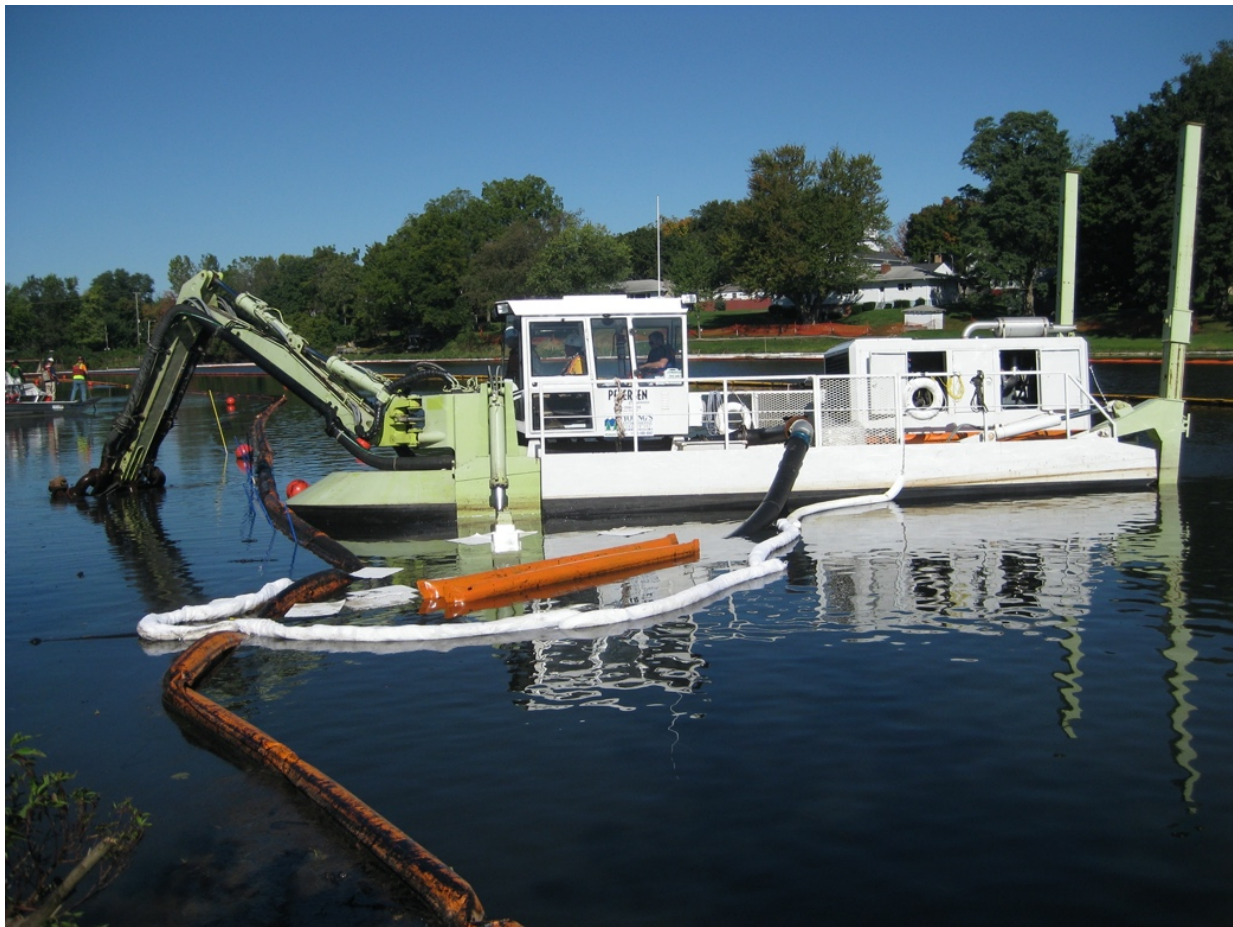
Figure 21. Integrated a hydraulic cutterhead dredge with a positive-displacement pump that was used during the response to the Enbridge Pipeline spill of diluted bitumen into the Kalamazoo River (USEPA, 2016).
