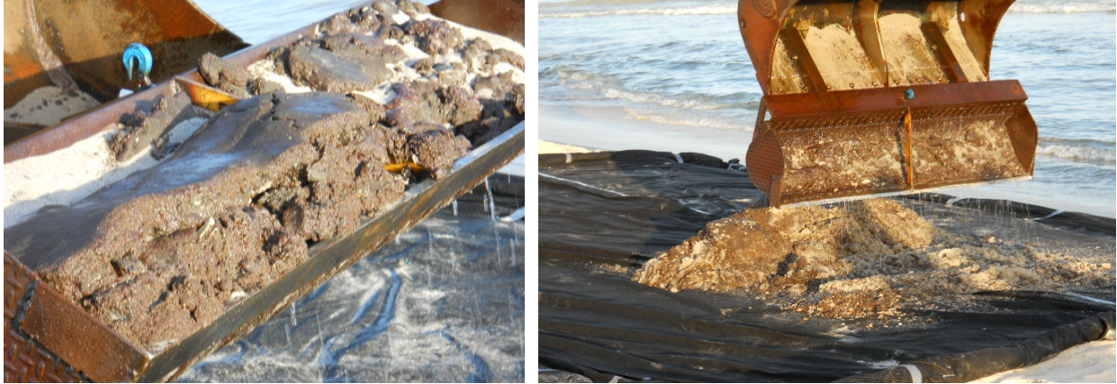
Figure 27. Long armed excavator removing SOMs along the Gulf coast during the Deepwater Horizon response. The excavator has a screened bucket welded to the front edge, which allows water and clean sand can drain out before the SOM material is placed on a tarp on the shoreline
