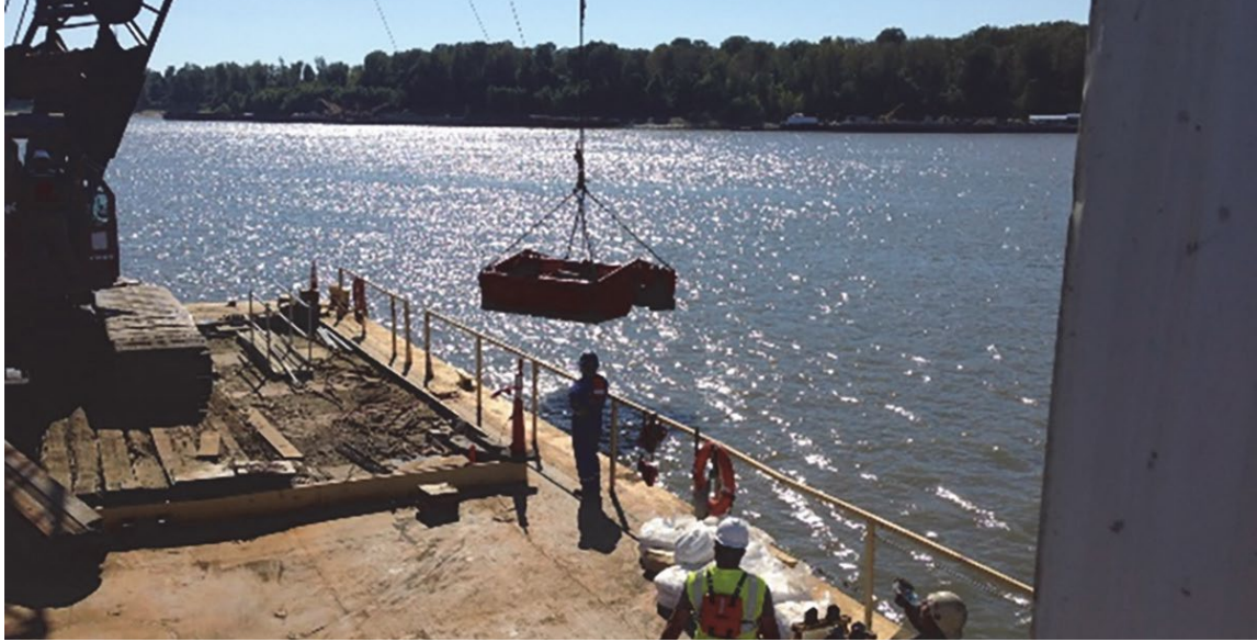
Figure 23. Environmental clamshell dredge used during the Apex 3508 oil spill response to recover sunken liquid oil (no SOMs present) in the Mississippi River.
