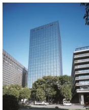
NBF Hibiya Bldg. (Chiyoda-ku, Tokyo)
