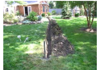
Trench for Coax
