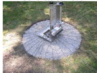
Radial Wires Installed Antenna Installed
