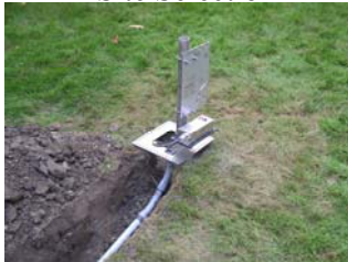
Coax to Base Install Radial Plate Tilt Base & VFCC
