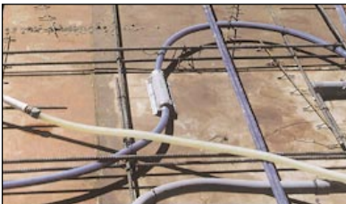
Stub Down Using Carlon's PV Mold
