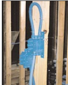
Wall Box Installation.
