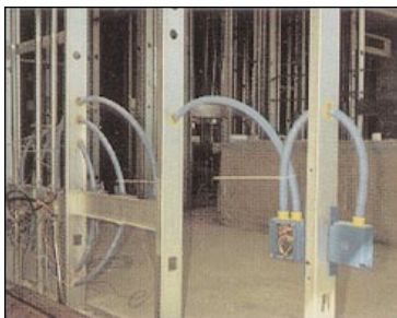
ENT installed in metal stud wall
