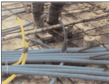
On Deck Installation – Hospital
