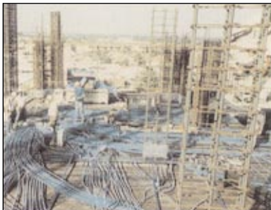
Slab On Grade
