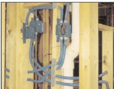
Wood Stud Installation – Condominium
