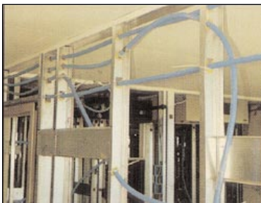
Metal Stud Installation – School
