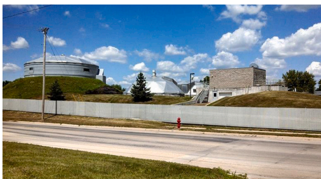
Detroit Lakes wastewater facility
