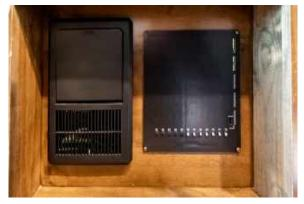
Figure 75.2 Wayfarer 12VDC Box Located Next to 12VAC Circuit Breaker Box in Bedroom Area of Motorhome
