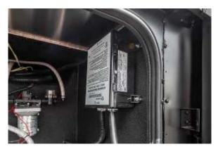
Figure 83.1 Automatic Transfer Switch
