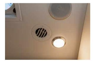
Figure 35.2 Roof Mounted Round Air Vent with Directional Air Guides Opened
