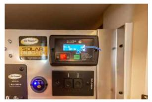
Figure 82.2 Remote Generator Start Switch Located on Central Control Panel
