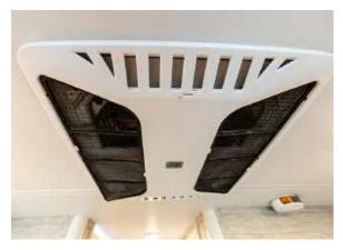
Figure 34.2 Chill Grill Covers Removed Exposing Vent Filters. Remove and Clean Periodically. Let Dry Before Reinstalling
