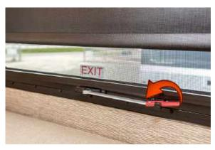
Figure 28.3 Lift Red Handle and Move Towards Left To Extend
