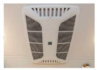
Figure 34.1 Roof Mount A/C with Chill Grill Vents
