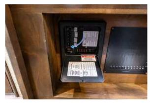
Figure 73.2 Wayfarer Breaker Box Located with 30AMP Main Breaker Highlighted by Blue Arrow
