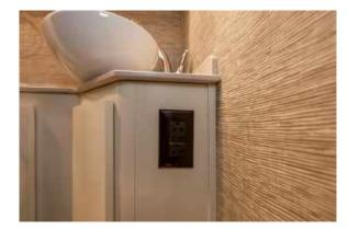
Figure 80.2 GFCI Receptacle Located in Bathroom Area
