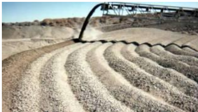
Figure 25 - Building a Stockpile using a Telescoping Conveyor
