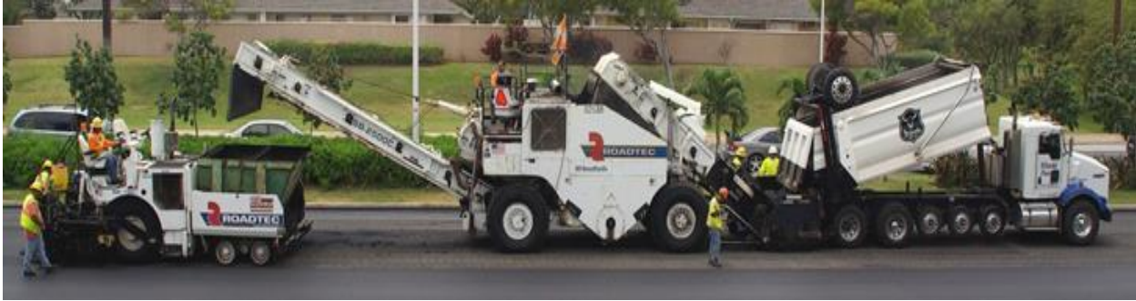
Figure 44 – Asphalt Paving Train
