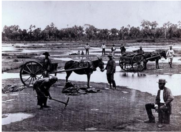
Figure 1 - Workers mining Trinidad Lake Asphalt
