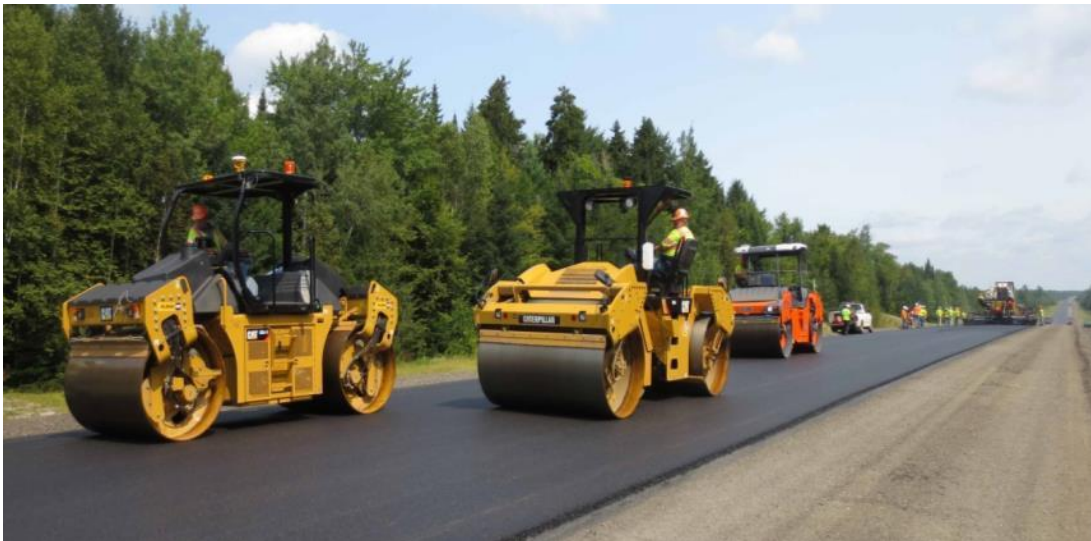
Figure 45 - Compaction Rollers
